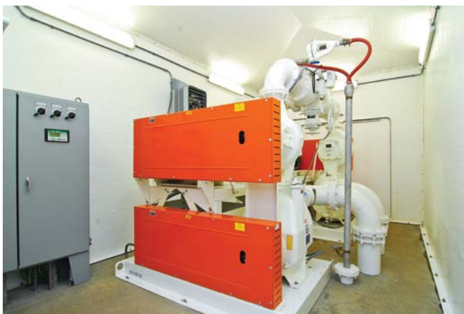
View of a complete set of Ultra-V pumps from the belt drive side. Photos courtesy of Stephen Vitosky.
